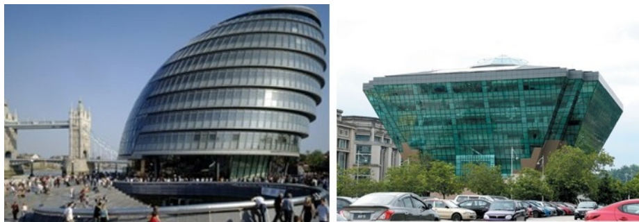
Figure 2: Self-shading buildings (left: London City Hall and right: Diamond Building in Malaysia)
